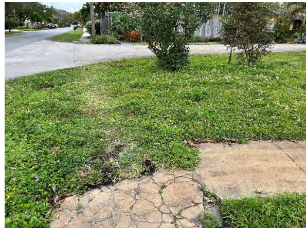
Incomplete residential sidewalk section on SW 17 th Street, west of SW 4 th Avenue.
