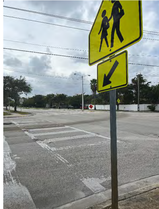
Faded pedestrian crosswalk at SW 4 th Avenue.
