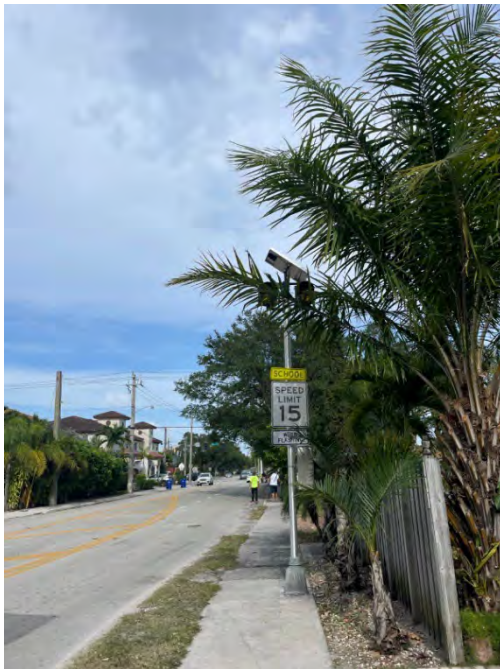
Observation 52: "Flashing lights are blocked by palm tree."
