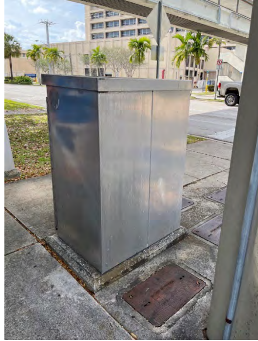
Observation 32: “Wrap Utilities in Art”
