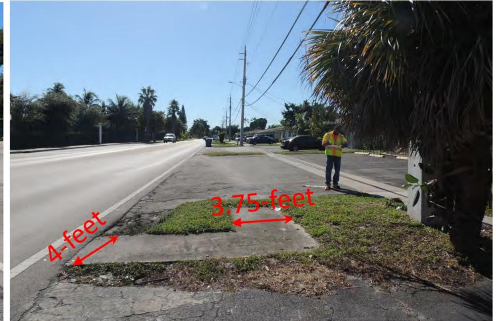
**Figure 225.2.1 Accessible Boarding and Alighting Area for Flush Shoulder Roadways with Connection to Sidewalk**
