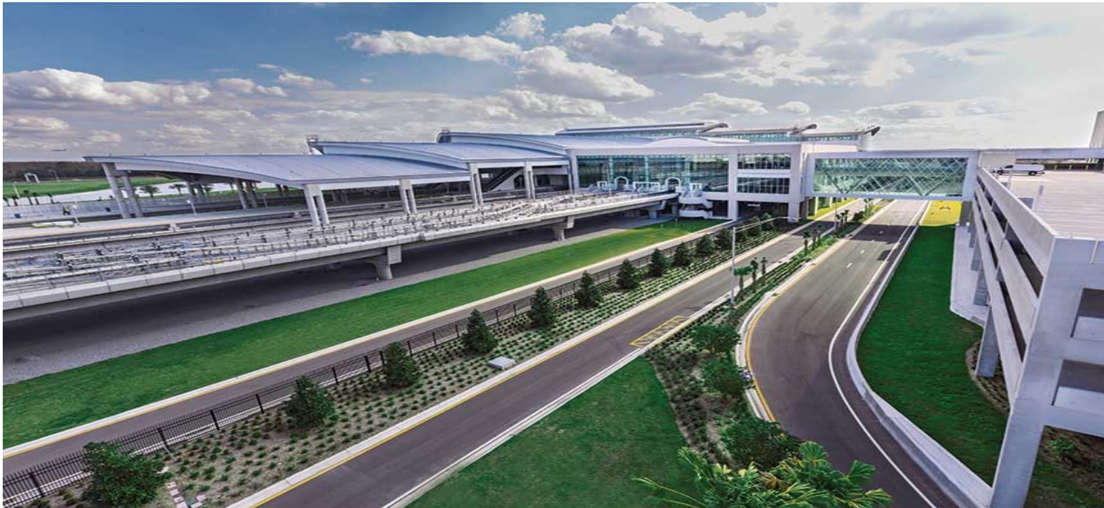
Orlando Station Complete
