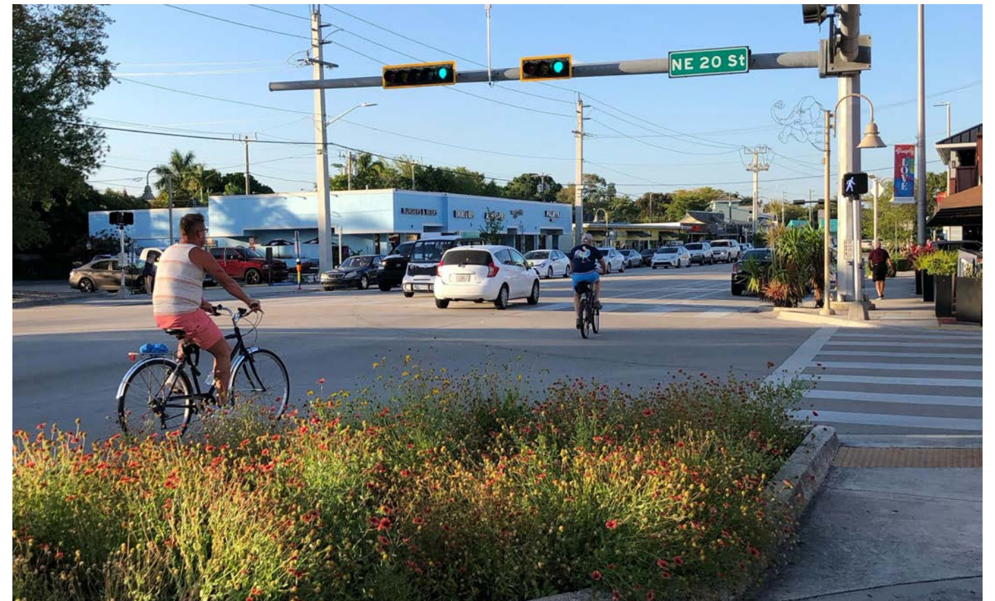
Bicyclists ride past native flowers in planters on Wilton Dr. The Wilton Dr lane reduction project also included marked bike lanes, decorative streetlights, high visibility crosswalks, and other complete streets improvements.
