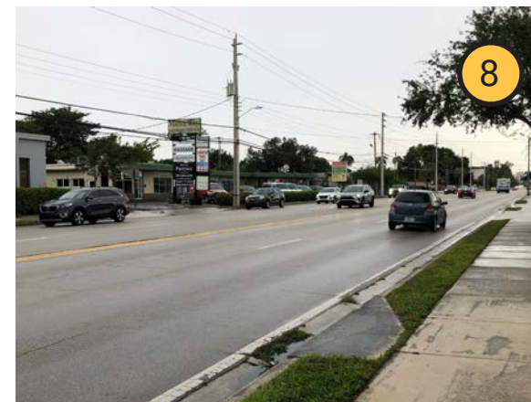
Continuous center turn lane plus numerous driveway openings can result in frequent turn movements.
