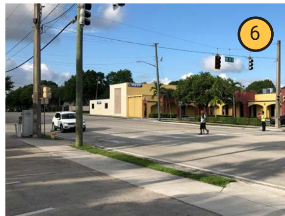
Crossing Guard assists crossing roadway; sidewalk abutting back-out parking and obstructed by mechanical equipment.
