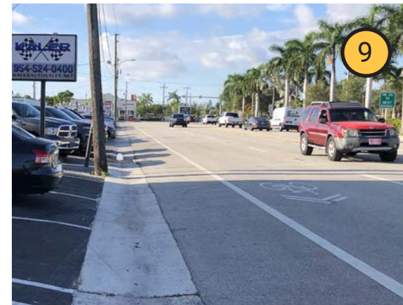
9 Sharrow markings on roadway with no sidewalk, back-out parking, and 5 travel lanes
