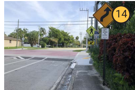
14 BCT Stop has sign only. RRFBs at raised intersection are single-sided
