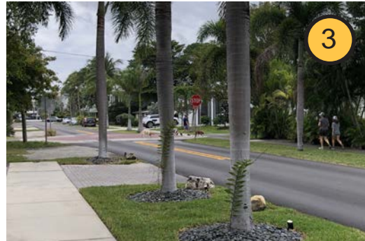
3 Sidewalk gap leading to raised intersection.
