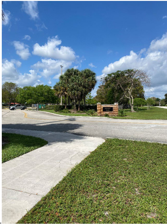
Gaps in sidewalks between Sunset Park and Hiatus Road
