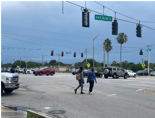
The marked crosswalk pavement markings at Southgate Boulevard and Rock Island Road/SW 71 st Avenue is faded.
