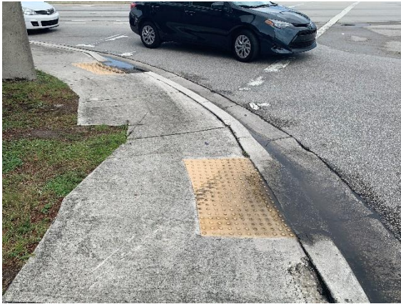
Drainage issues at the intersection of Southgate Boulevard and Rock Island Road/SW 71 st Avenue which causes pooling of water at curb ramps.
