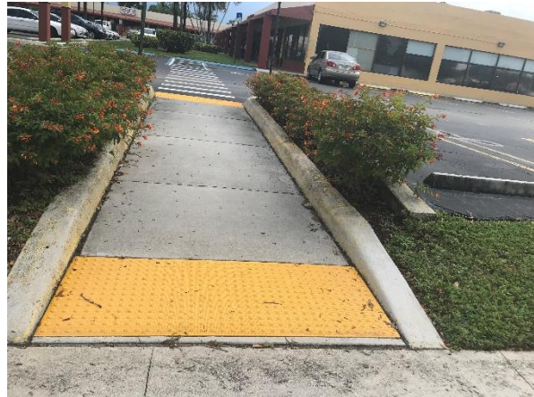
Several businesses along the corridor provide pedestrian access with ADA compliant detectable warnings and ramps. This access point leads to the Presidential Plaza shopping center.
