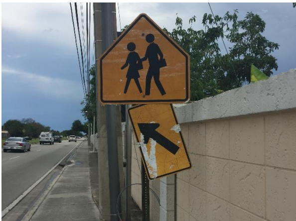
Pedestrian crossing signage damaged located at mid-block crossing along Southgate Boulevard east of SW 77 th Terrace.
