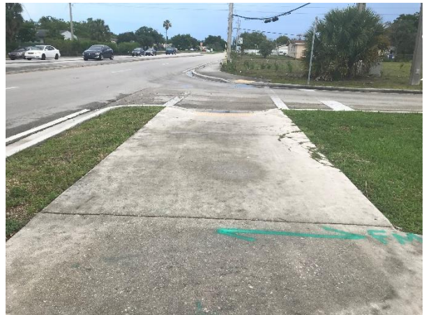
The pork chop island at the southeast corner of Southgate Boulevard and Rock Island Road/SW 71 st Avenue forces pedestrians to cross a lane of right-turning vehicles with no pedestrian signal.
