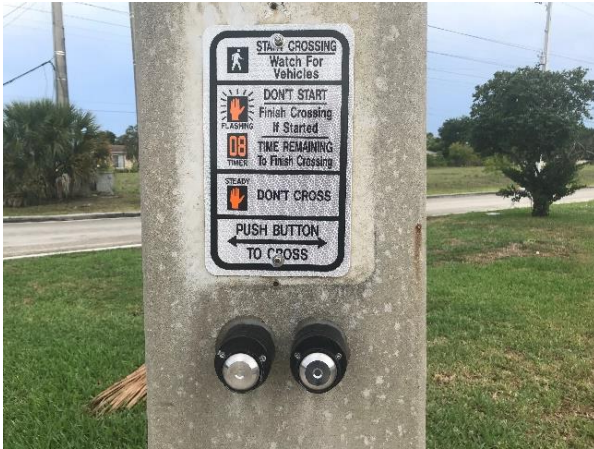
Pedestrian push buttons are not oriented toward desired crossing street and signage is not provided for each approach.
