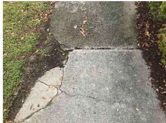
Sidewalk cracking which causes trip hazards.
