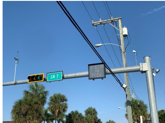
Variable message sign for NO TURN ON RED/YIELD TO PEDS on all four legs at the intersection of Southgate Boulevard and SR-7/US-441.
