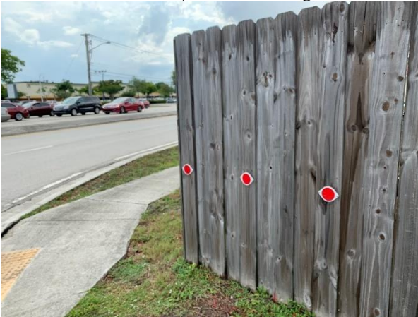
The wooded fences at the northwest corner of Southgate Boulevard and Rock Island Road may pose a visibility threat to motorists.
