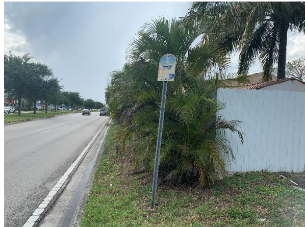
Route D stop located west of SW 73 rd Terrace does not have proper bus stop amenities such as ADA landing pad/passenger waiting area, bench, shelter, trash receptacle, lighting & etc.
