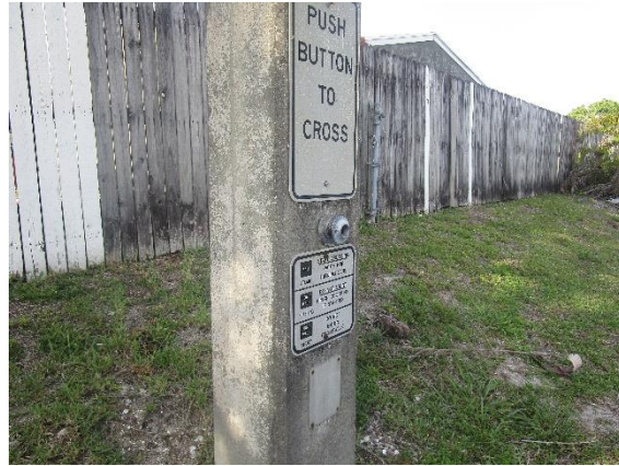
Outdated pedestrian pushbutton at mid-block crossing along Southgate Boulevard east of SW 77 th Terrace.
