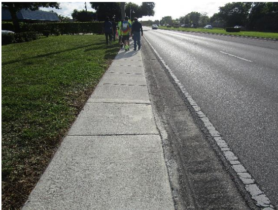
Curb cut for former driveway west of SW 75 th Terrace is unnecessary and should be reconstructed.
