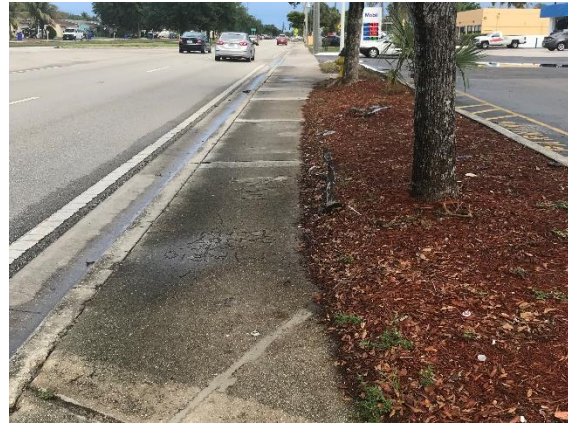
Unmaintained landscape encroaches the sidewalk facilities.
