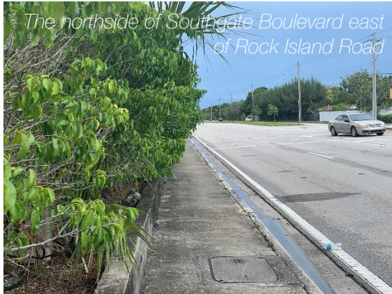
The northside of Southgate Boulevard east of Rock Island Road Overgrown trees endanger pedestrians and block the view of pedestrian signs.
