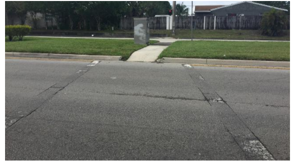
The mid-block crossing along Southgate Boulevard east of SW 77 th Terrace marked crosswalk pavement markings is faded and no detectable warnings.
