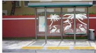
Bus Shelter with bench
