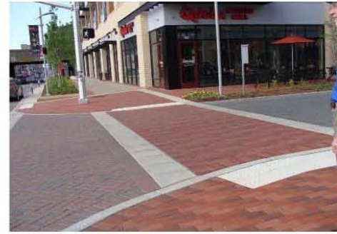
Raised Pedestrian Crosswalk
