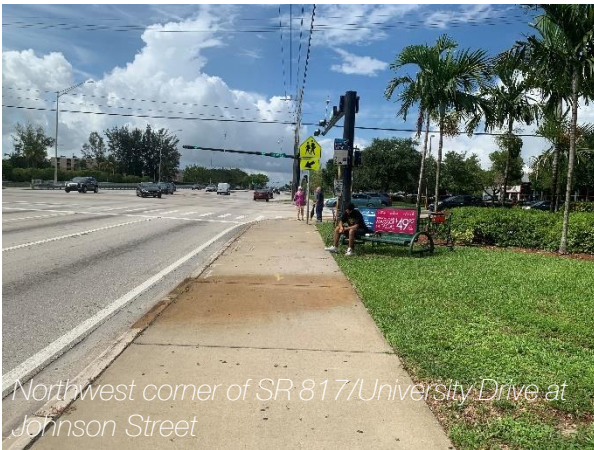
BCT Stop ID# 0299 does not have a hard surface concrete pad for the placement of the bench and is lacking amenities such as a shelter, bicycle racks, trash receptacles, etc.
