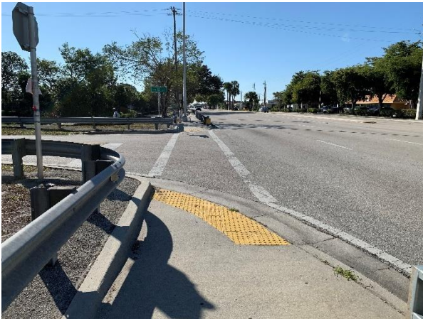
Marked crosswalk with detectable warnings on curb ramps is present at SR 817/ University Drive at NW 13 th Street which is an east-west road that leads to residential neighborhoods.
