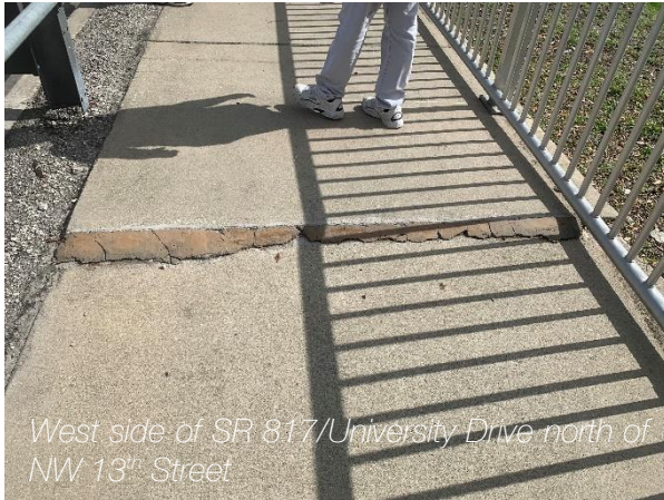
Cracked sidewalk/trip hazards along the sidewalk.
