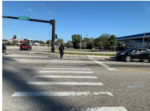
The intersection of Johnson Street and Taft Street has special emphasis crosswalk markings with pedestrian pushbuttons.
