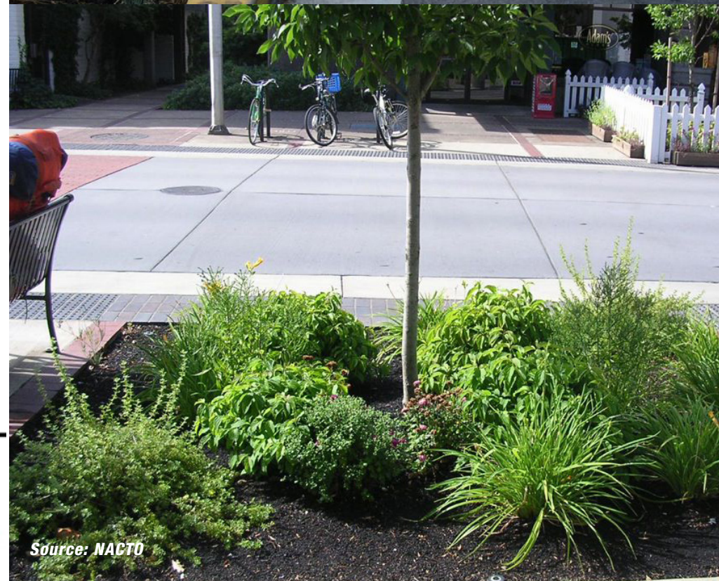
Bioswales installed at a mid-block crossing
